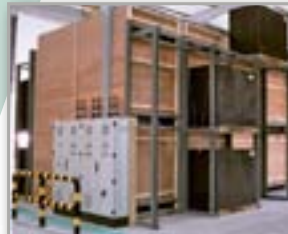
Installation for drying seed per box individually (open drying system)
